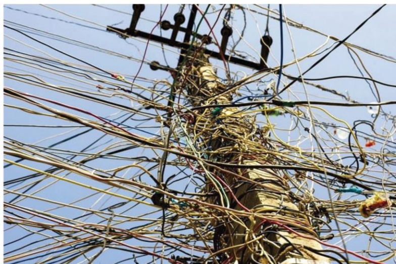
Figure 10 Electricity theft through unauthorised connections (photograph courtesy of Pradesh18, 2015)
