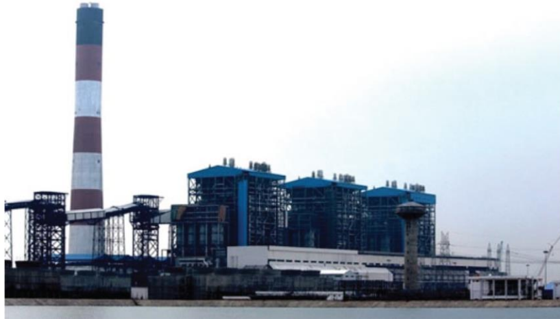
Figure 12 Lalitpur Super Thermal Power Project (STPP) in Uttar Pradesh (Lalitpur Power Generation Company 2016)
