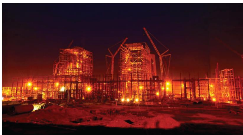
Figure 11 Tata Power UMPP at Mundra, Gujarat under construction (Tata Power 2015)
